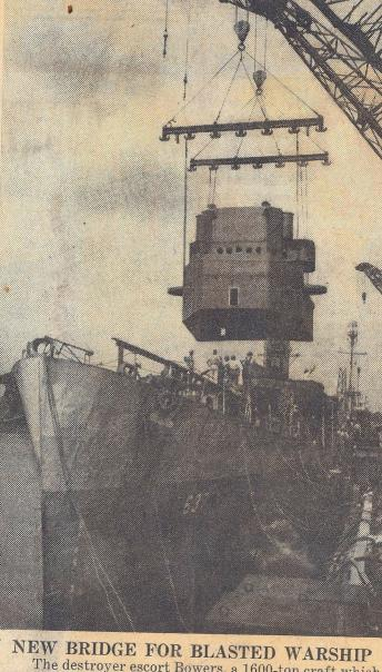
The destroyer escort Bowers, a 1600-ton craft which limped into the Philadelphia Navy Yard after being hit by a Japanese suicide plane off Okinawa, having a new bridge installed during the extensive repairs made here. Her crew of 200 suffered 105 casualties.
